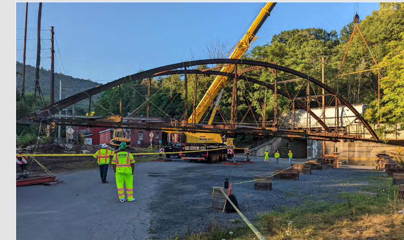
Two cranes lifted the 37,000 pound bowstring off its Mount Carbon abutments in 2022. After careful disassembly, an Ohio blacksmith transported pieces to his shop for rehabilitation. It was reassembled and placed on this trail in 2023.
